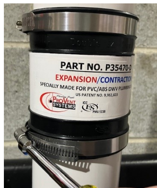
Tighten up the stainless steel bands 5
