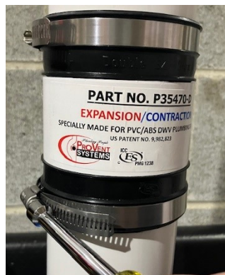
Tighten up the stainless steel bands 5
