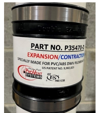
EZ Flex joint flexes vertical 6
