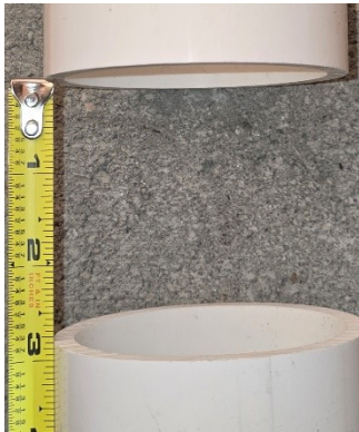
Leave a 2-3/4" gap between the pipes 1
