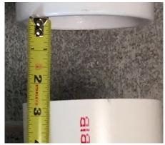
Insert a 2-1/2" gap between the pipes
