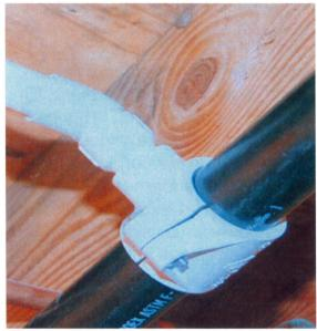
THE 1" DRAIN CAN BE CONNECTED TO THE NEARBY PLUMBING DRAIN USING A SADDLE TYPE CLAMP DEVICE INTO A PVC OR ABS PIPE OR THE DISCHARGE PIPE CAN BE RUN THROUGH TO AN OUTSIDE WALL.
