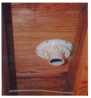
THE TRAP GUARD DRAIN IS MOUNTED FROM UNDERNEATH THE FLOOR USING CAULK AROUND THE FLANGE TO WATER-PROOF THE DRAIN THROUGH THE FLOOR.
