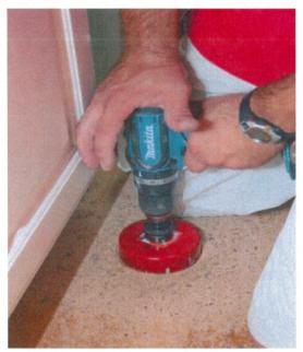
A 4" HOLE IS DRILLED THROUGH THE FLOOR AT A DESIRED LOCATION. IT CAN BE DRILLED IN A LOCATION OUTSIDE THE PLASTIC WASHER PAN OR UNDERNEATH THE PAN ITSELF.
