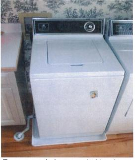
Emergency drain connected to a heavy duty washer pan protects against water damages throughout your household.
