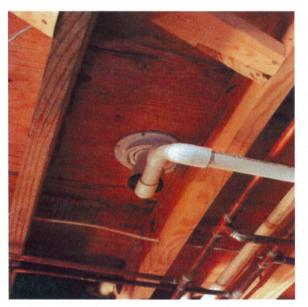
THE 1" PVC PIPE IS CONNECTED FROM THE PLUMBING LINE OR FROM OUTSIDE TO THE TRAP GUARD DRAIN TO COMPLETE THE INSTALLATION.
