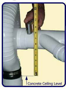
Make sure all the fabricated overhead piping will fit into the drop ceiling space. The stack sleeve can be raised up to recess the stack up into the slab if necessary. Drop ceilings are usually 12". Here we are 7-3/4" below the concrete ceiling.
