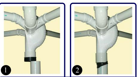
A rolled back E-Z Flex Coupling can be ordered solvent cemented into a PVC coupling at the factory. This allows inserting the stack pipe in-between the floor and the ProVent Stack fitting.
