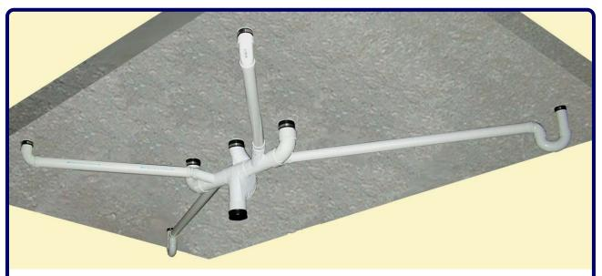
The embedded sleeve couplings also act as a hanger and riser clamp (see WH listing) for the horizontal and vertical piping. Additional hangers will be required if the branch piping exceeds the horizontal lengths allowed by code.
