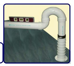
You will be fabricating upside down so the pitch on the pipe will seem like it's pitching the wrong way. It must pitch from the fixture openings back to the stack branches.
