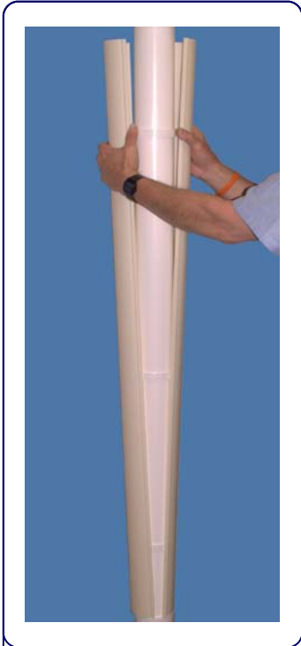
Place both halves of the Shell Pipe around the PVC pipe and rings
