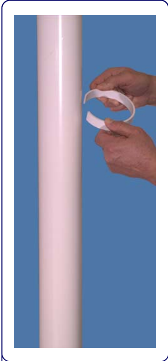
Install 2 ProVent PVC Spacer Rings around the existing PVC Pipe
