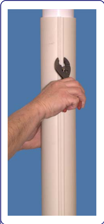
Snap the tongue of one half of the Shell Pipe into the groove of the other
